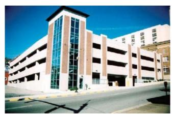
additional 20,000 sq. ft. of area on grade for a total area of approximately 70,000 sq. ft. The project entailed extensive use of thin-set brick panels and expansive glass in the main stair/elevator enclosure as its primary architectural features.
