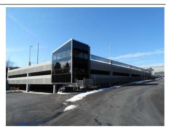
office/hotels that needed the parking support. CWC designed a two level precast concrete garage with independent entrances from each level reducing the need for integral ramps. The stair towers were encased in glazing to match the upgraded buildings throughout the facility and solar panels were eventually added to the roof of the garage.
