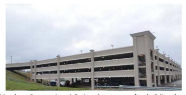
Project Description: CWC was contacted by the Meadows Racetrack and Casino three years after building the original garage in 2009 that was connected to the casino. This second garage was delivered in the design/build system as well and was a stand-alone structure to help support the casino's massive growth and development. CWC designed a precast superstructure with cast-in-place concrete elements and a façade that matched the original garage and casino development.
