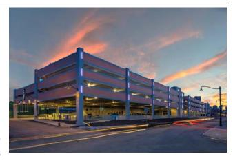
Development. The garage is centrally located to the entire development to support the new living and office space throughout the development. The garage was designed with deep foundations, a precast superstructure and a cast-in-place topping on the second floor to protect the retail developments below. The façade consisted
