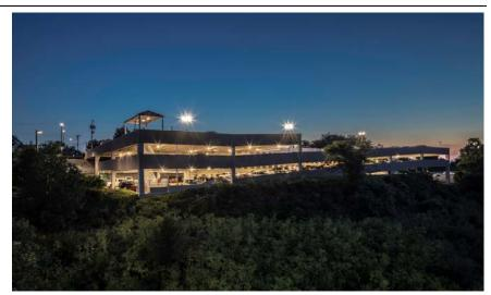
Hospital. The project was built utilizing deep foundations, precast concrete, with brick stamped spandrel panels to match the hospitals aesthetic. The garage took advantage of the existing topography to include multiple levels of entrance and exit to help eliminate congestion during high turn-over shift changes. The garage was completed on time to allow the hospital to further expand their hospital facility.
